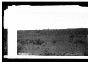
5261 QUERETARO, THE OLD ACQUEDUCT
