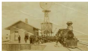
5201 STATION OF SAN JOSE
