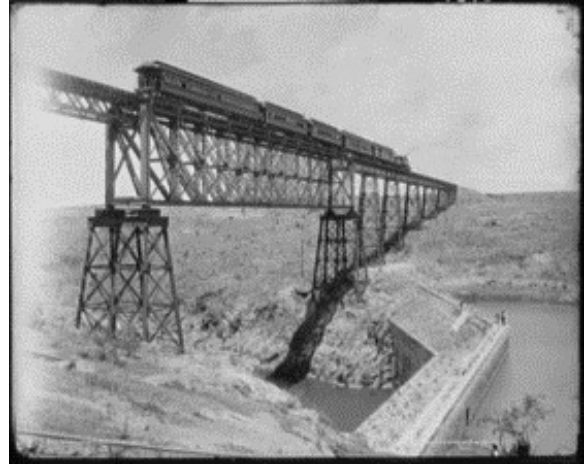
1610. BRIDGE NEAR ENCARNACION, MEXICO (18x22") 475
